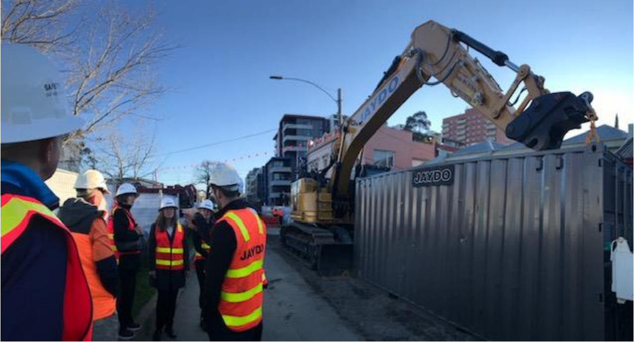
Photo 1: CRG group tour around M205 stage 1 construction site.
