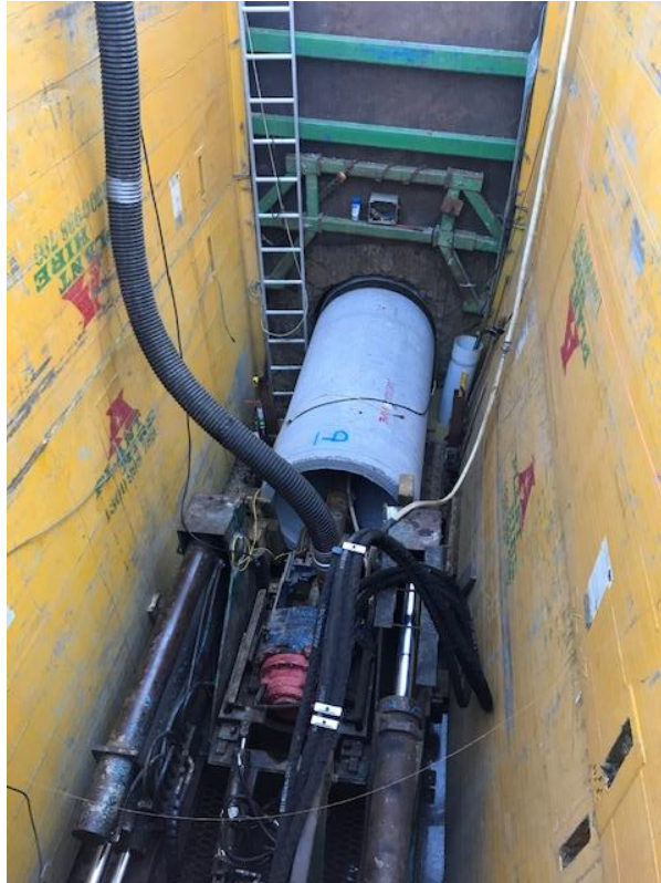
Photo 3: Micro Tunnelling Bore Machine (MTBM) view from the launch shaft.
