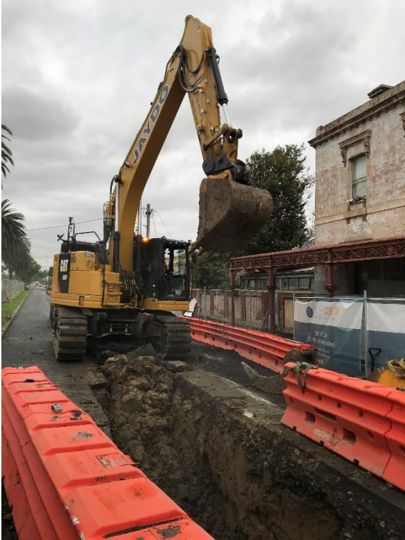
Image 4: 35t excavator digging trench.
