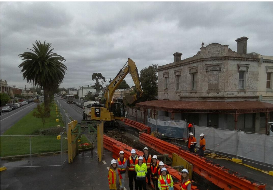
Image 6: CRG at trenching site
