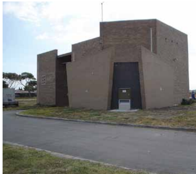
Raw sewage enters the plant.
