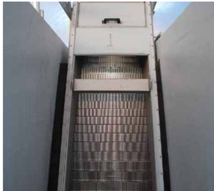
Cotton buds, bits of plastic and debris are removed from the sewage.
