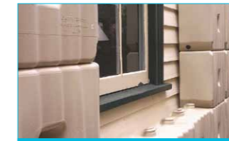
Modtank stored along the wall.
